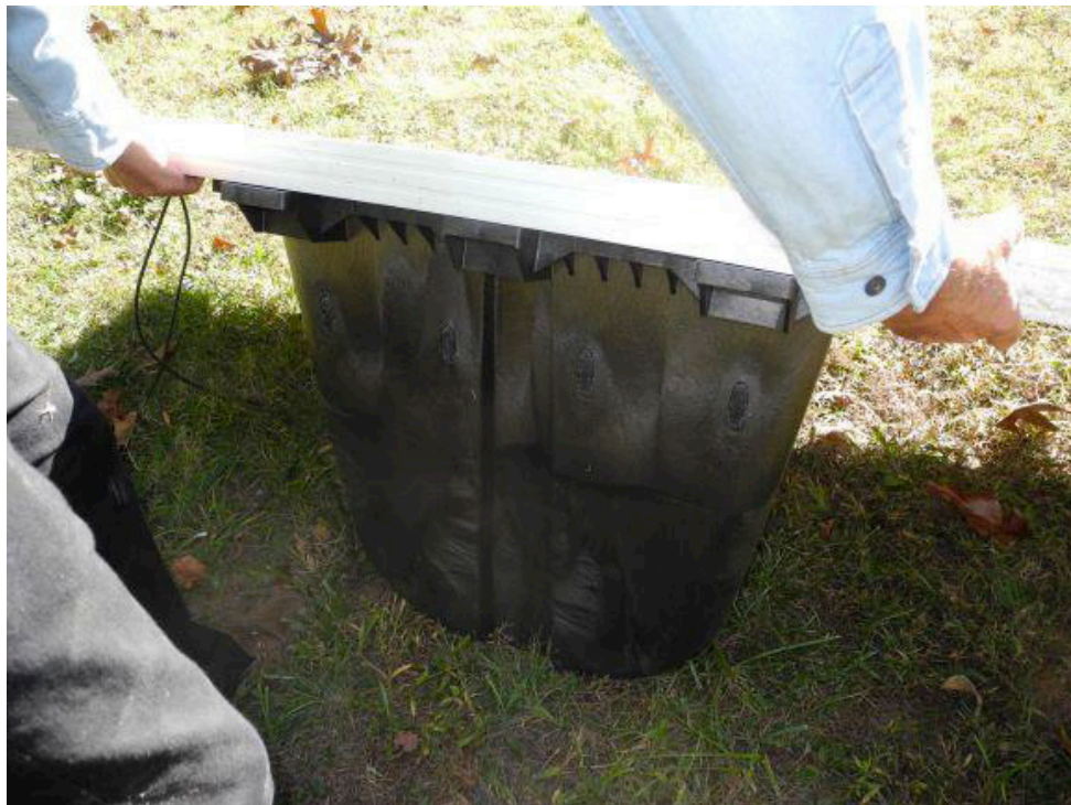
Figure 14. Panel resting on tabs ready to slide down to seat panel frame flanges in slots.
