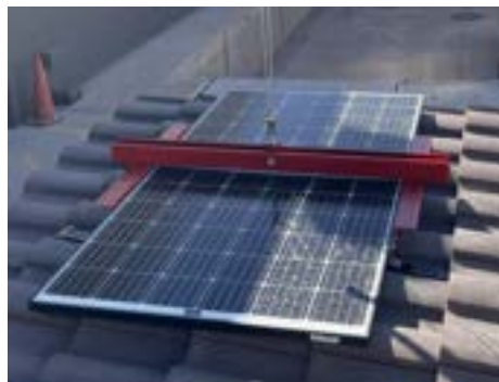
PHOTO 2: Overview of tensile test setup and connection
