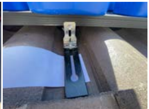
PHOTO 6: Load 2 - Bracket under load
