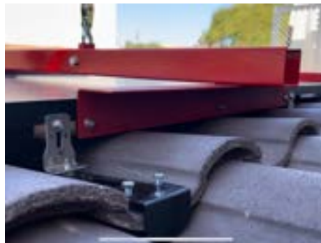
PHOTO 8: Bracket unloaded after test
