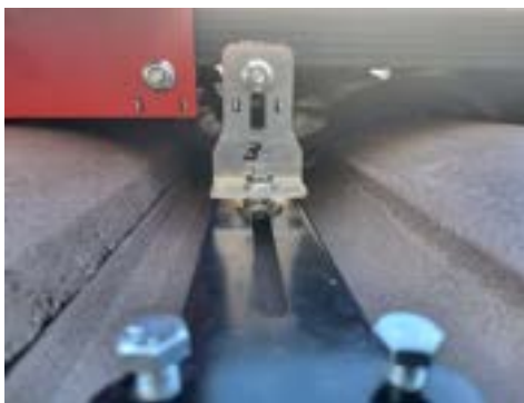
PHOTO 2: Typical Bracket - before tests
