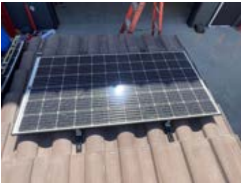
PHOTO 1: Overview of solar panel and tile roof deck - before tests
