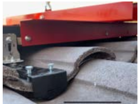
PHOTO 7: Bracket under test load
