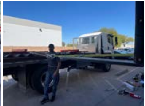
PHOTO 3: Test setup for horizontal pull load
