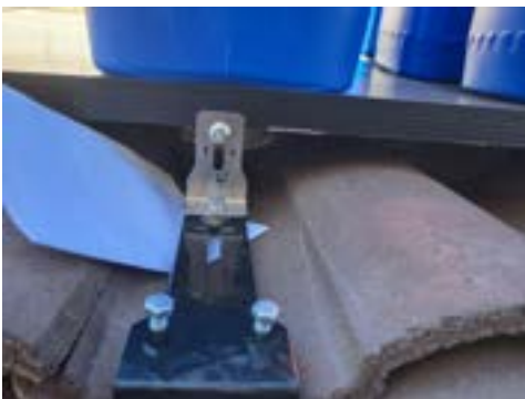
PHOTO 4: Load 1 - Bracket under load
